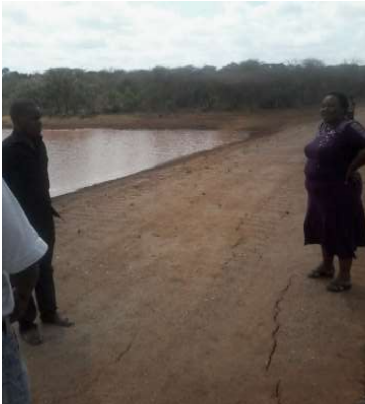
Figure 2 A complete Winzyeei earth dam
