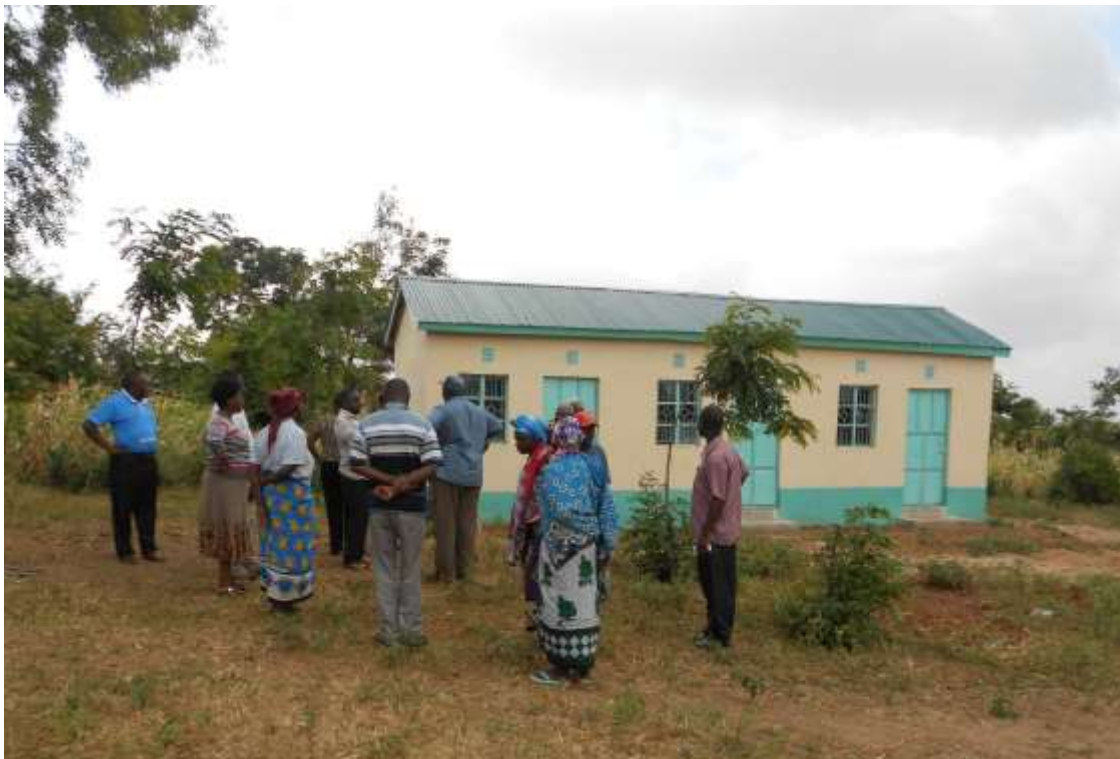
Figure 1 Inspection of Kitungati AP line
