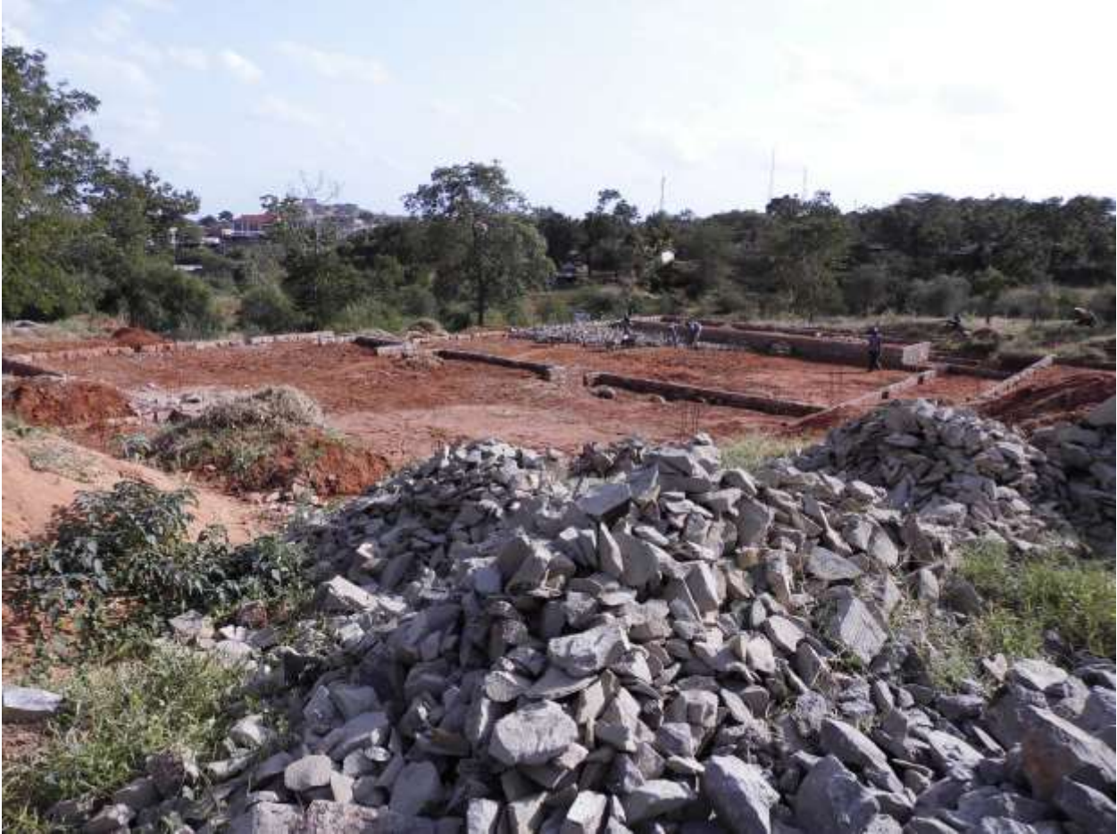
Fig 8. Site of the Mwingi Resource centre under construction.
