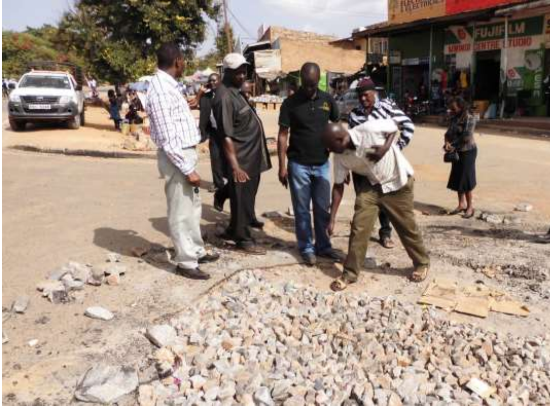
Figure 12 Inspection of Mwingi Town road carpeting
